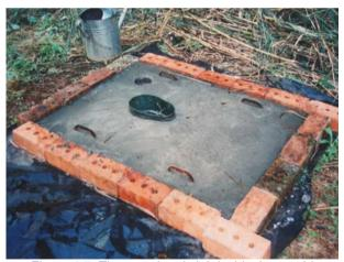
Figure 4-7: The completed slab inside the mould
