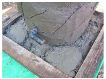
Figure 6-23: Wire added for reinforcement
