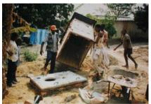
Figure 7-10: Fossa alterna built on a rectangular slab
