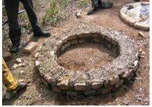
Figure 3-12: Completed brick ring beam
