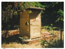
Figure 4-1: A portable structure using poles and reeds
