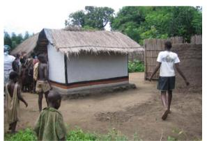
Figure 4-3: A permanent structure housing both pits
