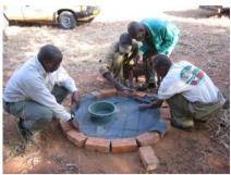
Figure 3-41: Laying down reinforcement wires
