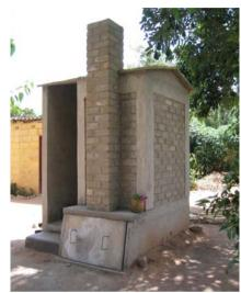
Figure 6-42: A brick single-vault urinediverting toilet
