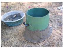
Figure 6-20: Concrete added half-way up the bucket
