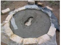
Figure 3-9: Mould after removal of squat hole insert
