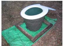
Figure 6-22: Bucket and seat turned over and placed into base mould
