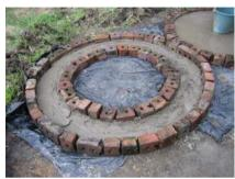
Figure 3-30: Concrete mix added to mould
