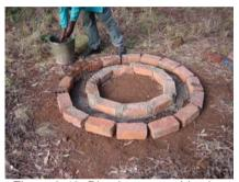
Figure 3-43: Ring beam mould using bricks
