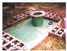
Figure 6-2: The brick mould for the toilet slab
