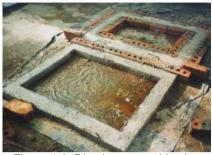
Figure 4-9: Ring beam mould using bricks
