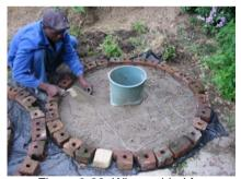
Figure 3-26: Wires added for reinforcement
