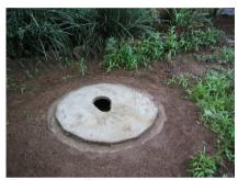
Figure 3-20: Toilet slab placed on ring beam
