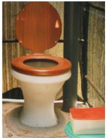
Figure 6-35: Urine-diverting pedestal with a handsome wooden seat
