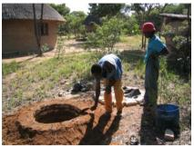
Figure 3-34: Packing soil around the brick ring beam
