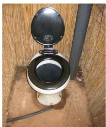
Figure 7-12: Fossa alterna upgraded with a urine-diverting pedestal
