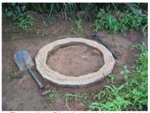
Figure 7-3: Ring beam laid on level ground
