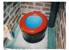
Figure 5-6: Finished concrete pedestal
