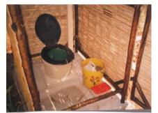
Figure 4-18: Inside a Fossa alterna that has been fitted with a pedestal
