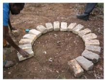
Figure 3-10: Forming the brick ring beam
