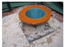
Figure 3-52: Low-cost pedestal on top of slab
