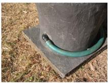
Figure 6-27: Urine outlet pipe attached
