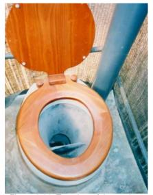
Figure 6-36: Top-view of the a urinediverting pedestal
