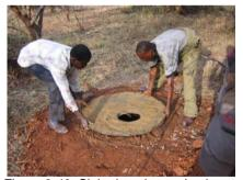
Figure 3-49: Slab placed over ring beam
