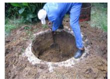
Figure 3-36: Digging the pit inside the concrete ring beam
