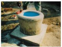
Figure 5-5: Painting the concrete pedestal
