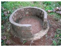
Figure 7-4: Brick wall built-up on ring beam
