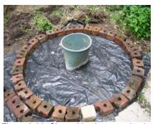
Figure 3-23: Shaped bucket to make the squat hole
