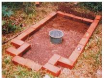
Figure 6-1: The brick mould for the base slab
