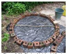
Figure 3-22: Circle of bricks 1.15m in diameter
