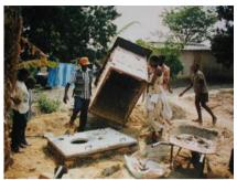
Figure 4-19: Fitting a portable superstructure to a Fossa alterna pit
