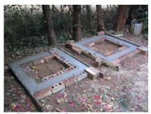
Figure 6-47: Casting ring beams
