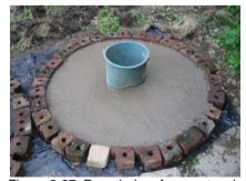
Figure 3-27: Remainder of concrete mix added and levelled-off
