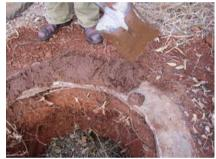
Figure 3-48: Anthill mortar packed around ring beam
