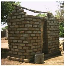
Figure 4-28: Brick double pit composting toilet
