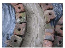
Figure 3-31: Wire reinforcement added
