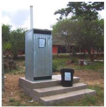
Figure 4-27: Fossa alterna with a metal structure
