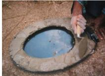
Figure 5-8: Plastic toilet seat filled with strong concrete
