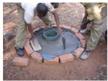
Figure 3-42: Levelling-off the concrete mix
