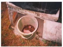
Figure 6-43: Removal of bucket of faeces
