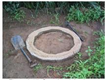
Figure 3-17: Completed ring beam
