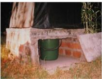
Figure 6-40: Internal view of vault with plastic bucket placed for collection of faeces
