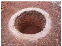
Figure 3-46: Pit dug inside ring beam
