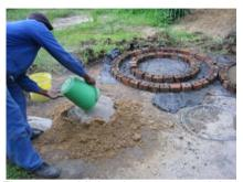
Figure 3-29: Mixing the cement and river sand
