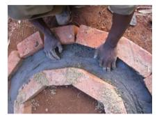
Figure 3-44: Addition of wire for reinforcement
