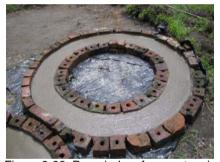
Figure 3-32: Remainder of concrete mix added and levelled-off
