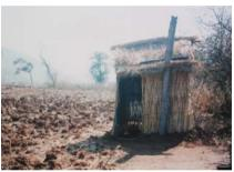
Figure 3-56: Another style of structure with a ventilation pipe
