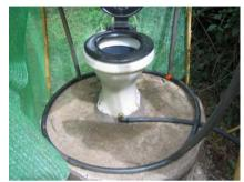
Figure 7-8: Urine-diverting pipe attached to base of pedestal
