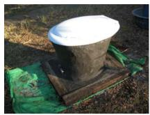
Figure 6-24: Completed pedestal curing
