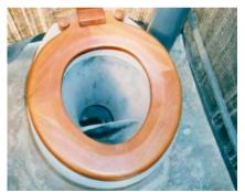
Figure 7-13: Urine-diverting pedestal mounted above the ground
