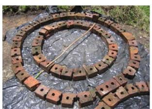
Figure 3-28: Two brick circles for ring beam mould
