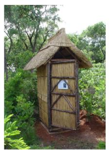
Figure 3-1: Simple compost toilet built on rectangular slab
