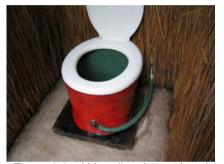
Figure 6-31: Urine-diverting pedestal installed
