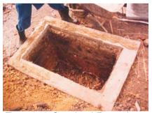
Figure 4-12: Completed Fossa alterna pit
