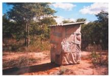
Figure 7-9: Arborloo built on a rectangular slab
