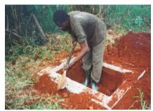
Figure 4-10: Digging the pit for the Fossa alterna
