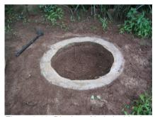
Figure 3-18: Digging of hole inside ring beam
