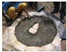
Figure 3-8: Cement and reinforcing wires in mould
